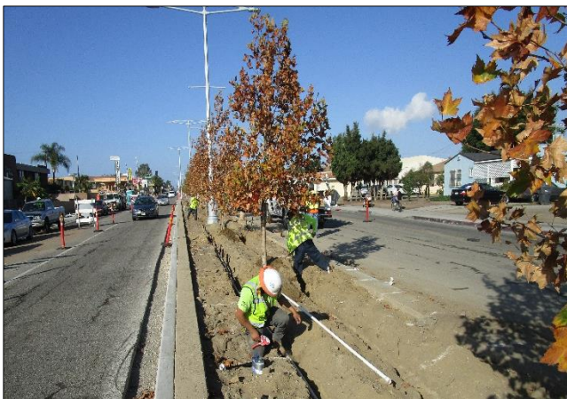
Installing Irrigation Laterals, Risers and Heads in Median
