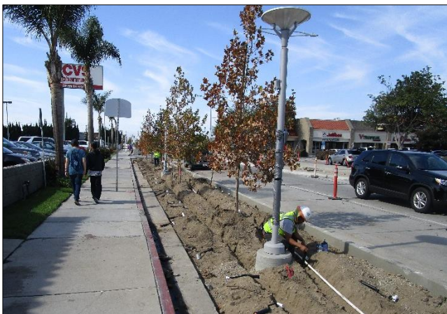
Installing Irrigation Laterals, Risers and Heads in Parkway
